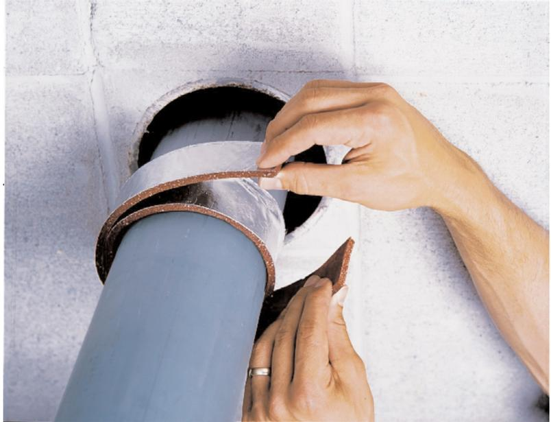
supporting. Applications include: telephone cable, metal pipe, plastic pipe, conduit, insulated metal pipe and cable trays. They can be used to firestop up to 10 inch (254,0 mm) diameter PVC pipe and are UL-Classified for use on PVC, CPVC, ABS, CCPVC, CCABS, PVDF, FRPP, PP and PB plastic pipe.
