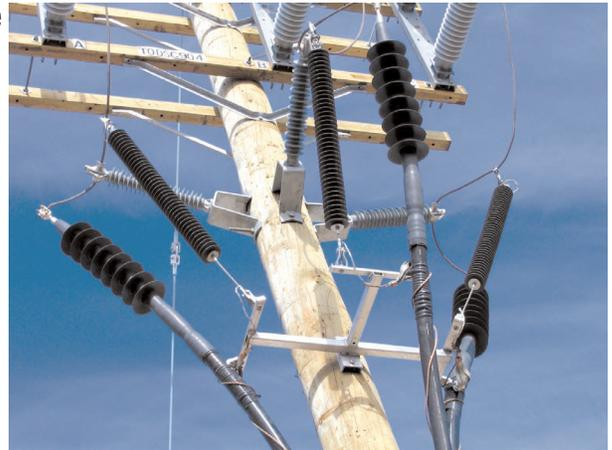
The QT-III terminations meet or exceed the requirements of IEEE 48, Class 1, 69 kV and IEC 60840 for 72,5 kV. The QS-III joints meet or exceed the requirements of IEEE 404, for 69 kV and IEC 60840 for 72,5 kV.
